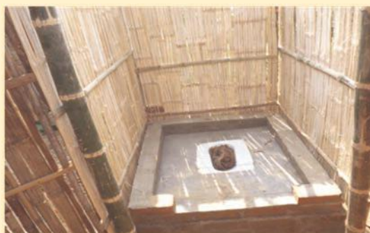
Newly constructed toilet at Fatuwa Mahespur VDC, Rautahat district
